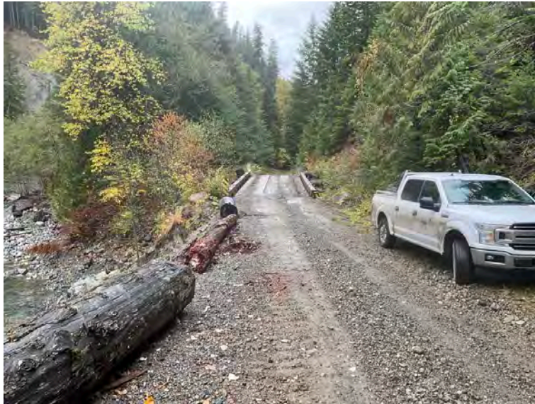
Approach from Left Bank when facing downstream
