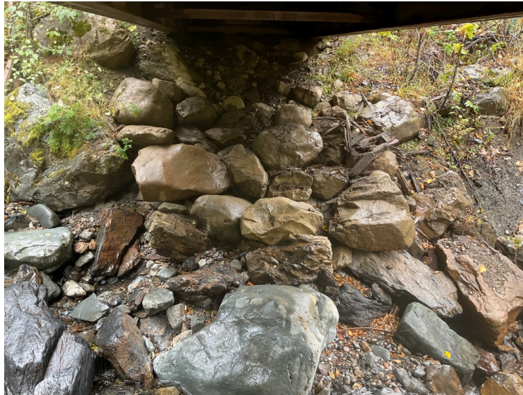
Left Bank Abutment when facing downstream
