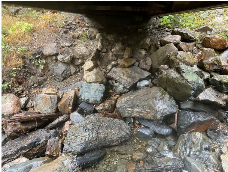
Right Bank Abutment when facing downstream
